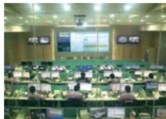
▲ Integrated Control System
